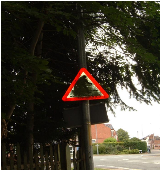
Example of advanced directional sign obscured by overhanging vegetation
