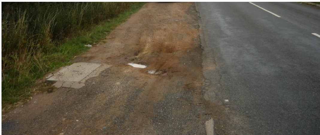
Example Lay-by on rural road that is unsigned and unsurfaced.
