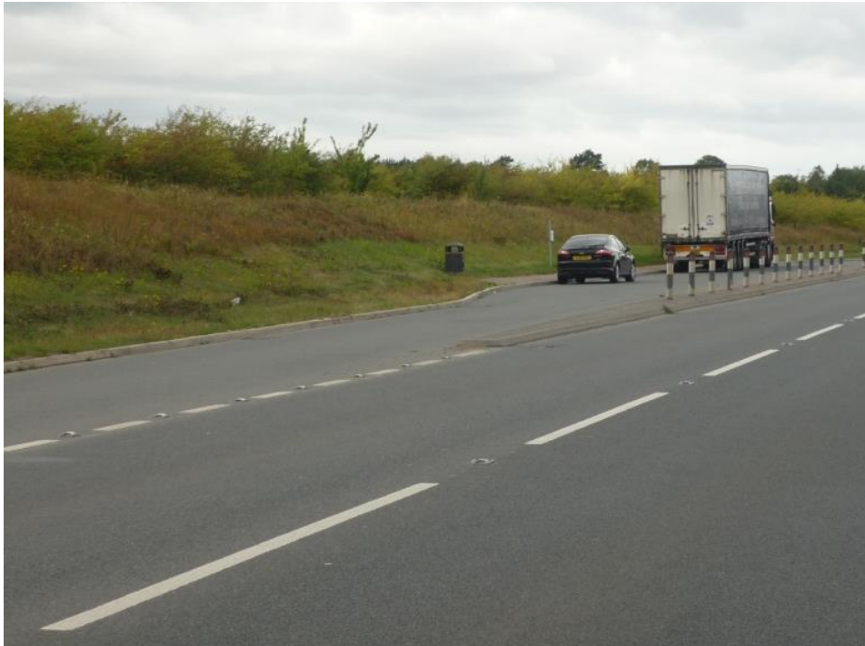
Purpose built Lay-by on the A44 Surface, signed and with a footway.
