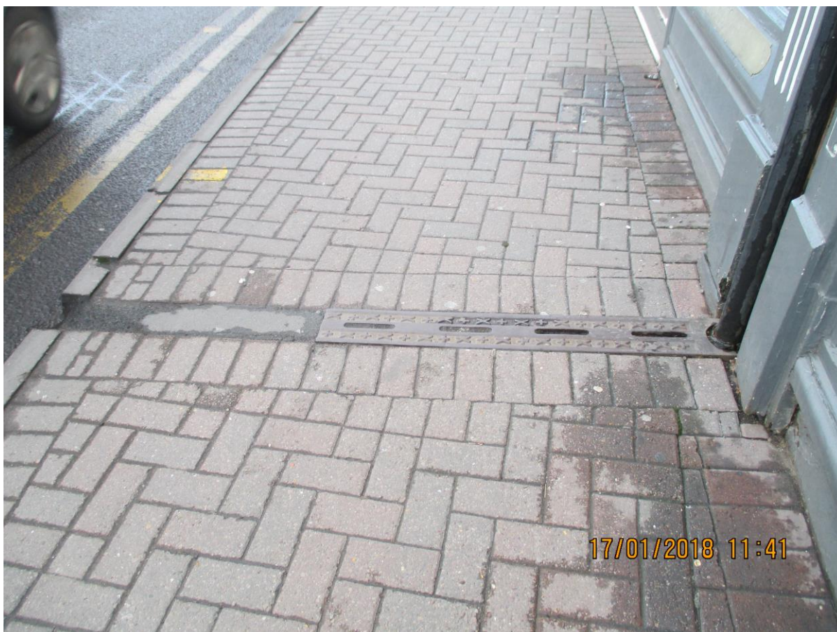
Example of Cross Footway Drainage Channel
