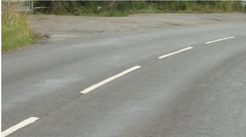
Example of a lay-by on rural road that is unsigned but stone surfaced
