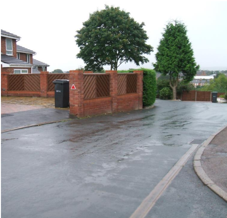
Example of wall built over an adopted service strip
