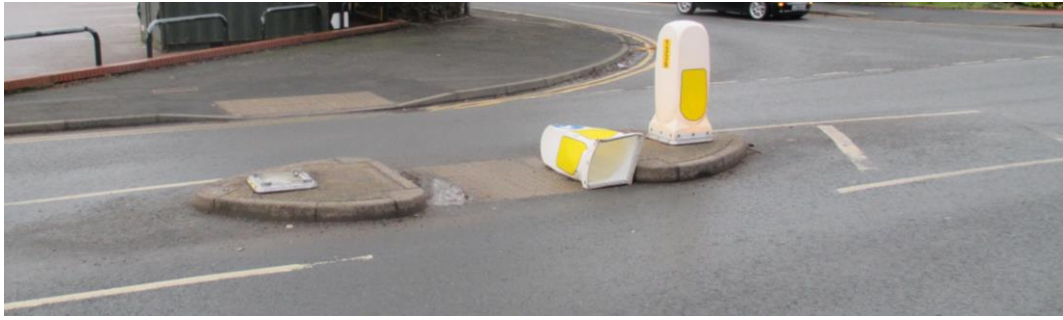
Example of illuminated traffic bollards
