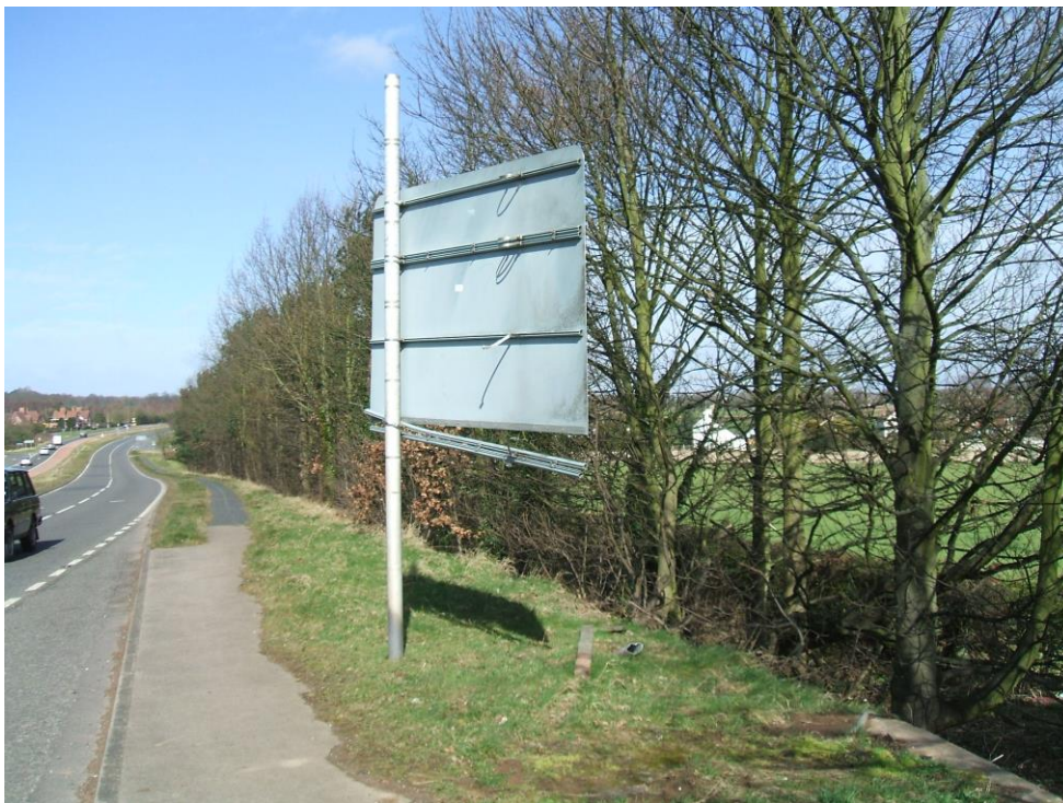
Example of accident damaged ADS
